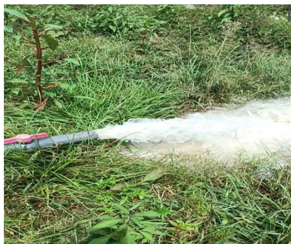
Fig 2. Wastewater effluent discharge point
